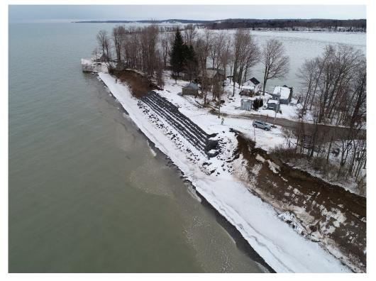
Figure 4-2 Recently constructed gabion wall
