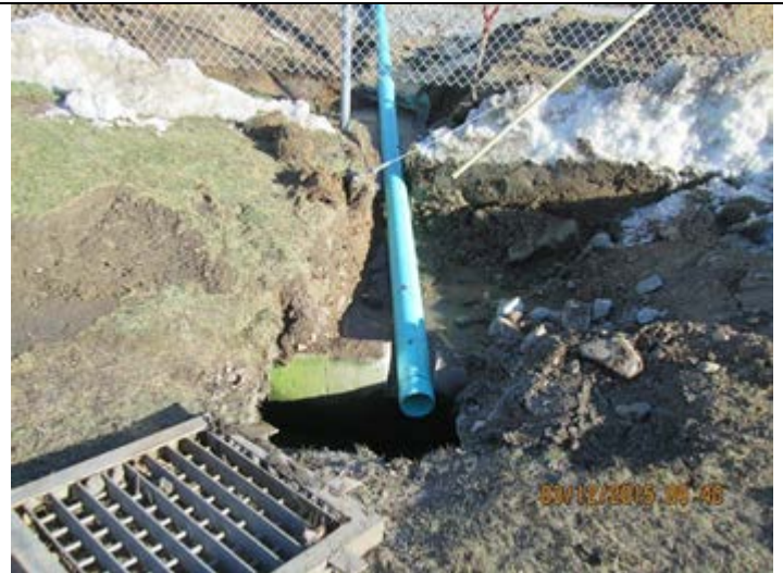
Outlet pipe from rain garden.
