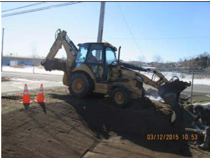
Placing stone and soil.
