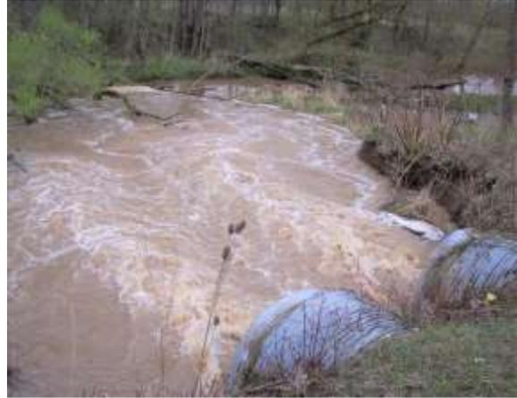
The severely corroded and damaged culvert located at the end of Gansz Road East only provides a conduit for the Canal to overflow into the Clyde River during the Canal's open season. The canal flows through the culvert until the river's inlet and outlet are equal with the water level equilibrium of the Canal. It does not contribute to the flow regime of the Clyde River, but uses the river as a backwater wetland. During the Canal's low water times, the River actually drains into the Canal.
